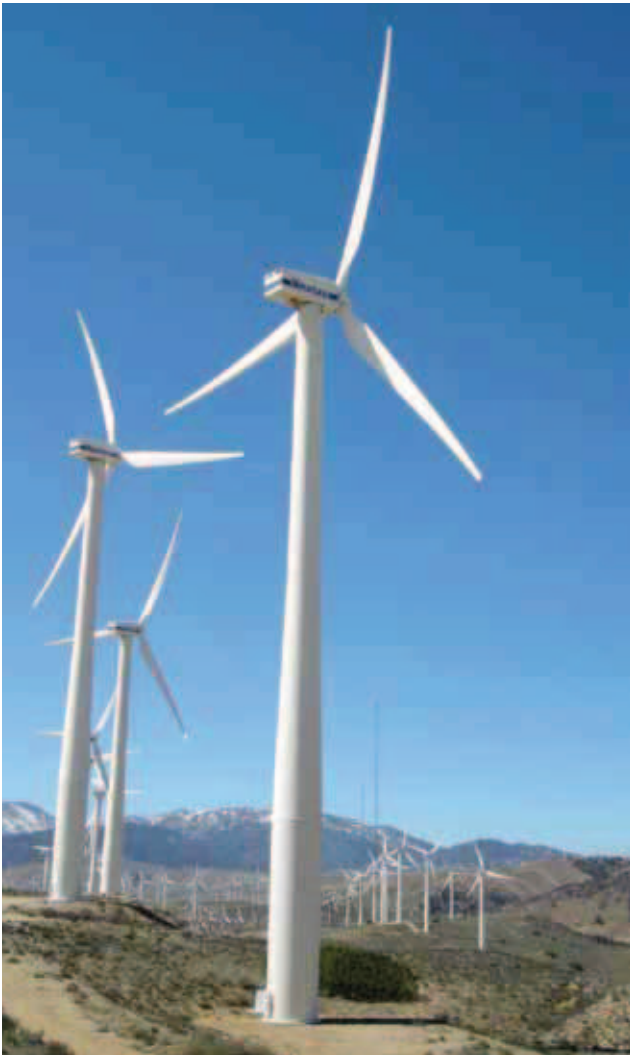
Wind power plant
